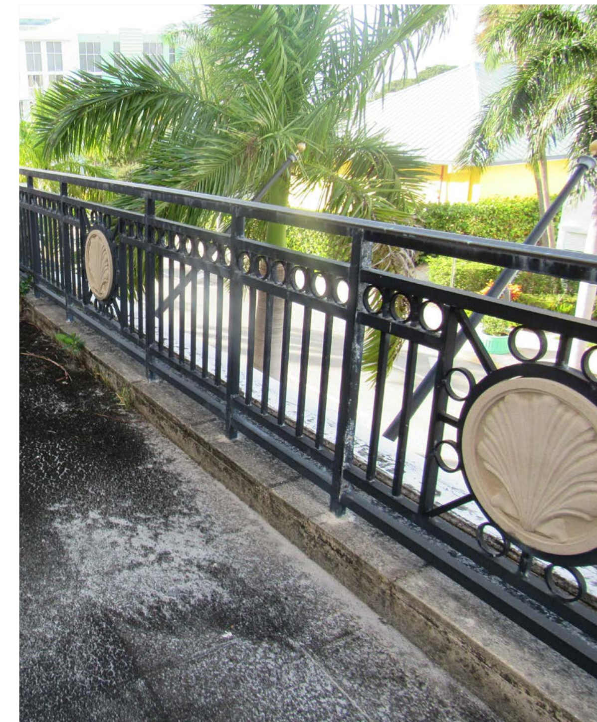
EXTERIOR METAL RAILINGS
