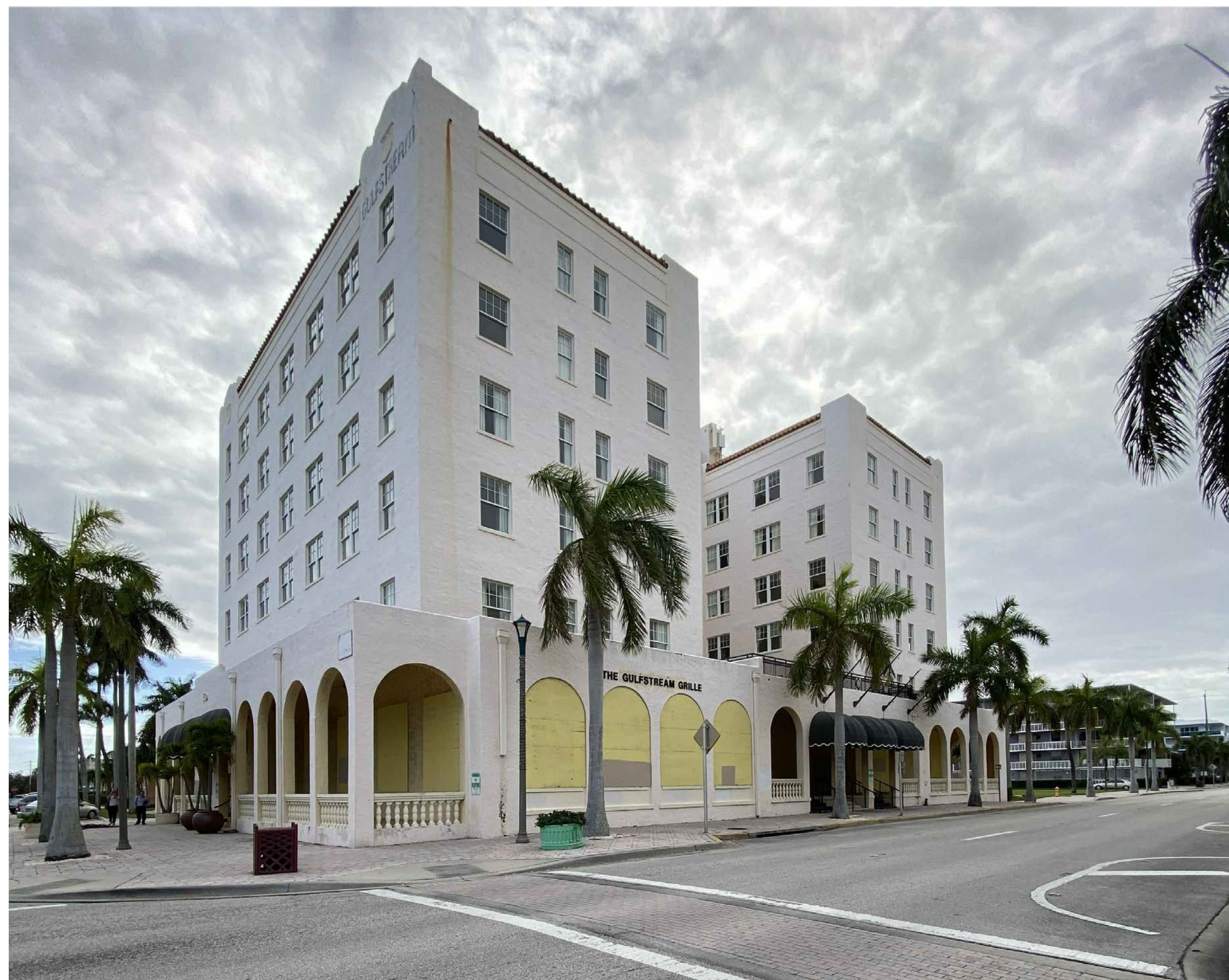
EXISTING BUILDING LOOKING SOUTHWEST ARCADE, DECORATIVE PARAPET, TRIMS, RAILINGS, TILE ROOF, SHIELDS AND SIGNAGE TO REMAIN. EXISTING WINDOWS AND DOORS TO BE REPLACED WITH NEW WINDOWS AND DOORS (MULLION CONFIGURATION TO MATCH EXISTING)
