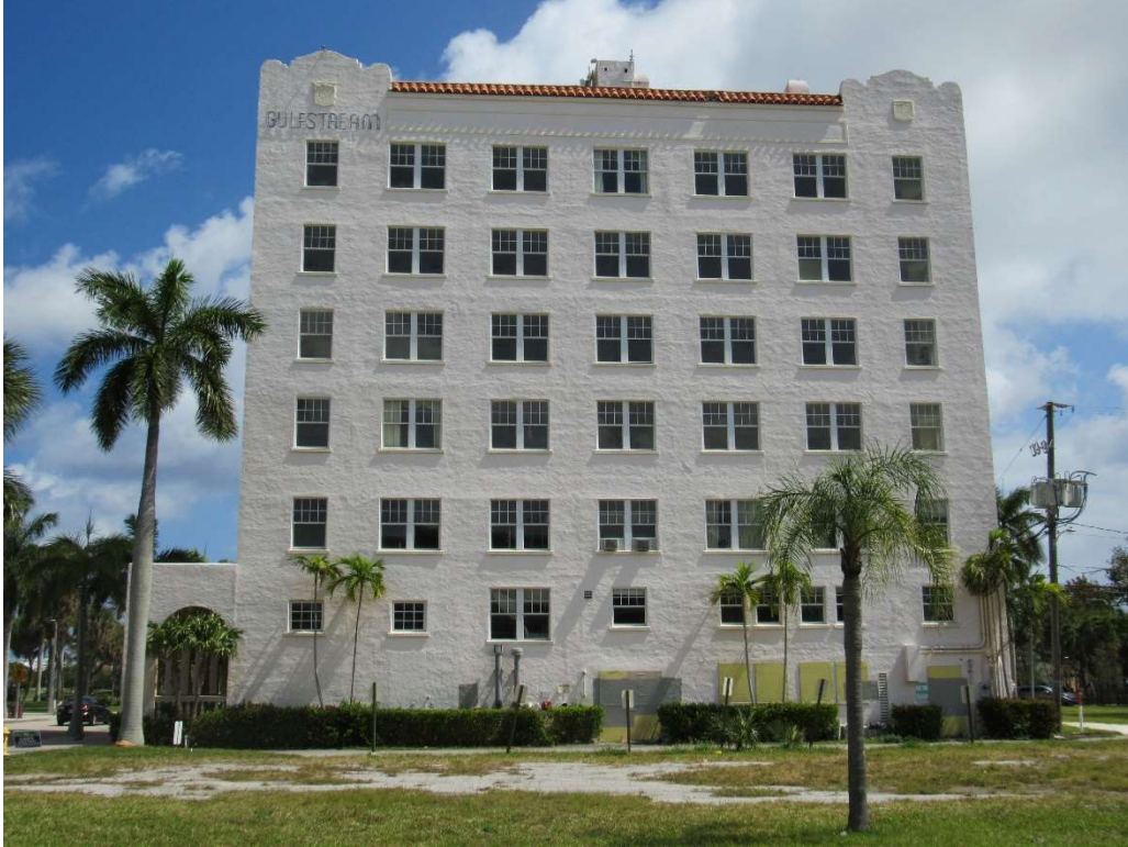
Photo #5 Gulfstream Hotel Building 1 Lake Ave, Lake Worth, FL 33460 View of W Elevation (3/12/2020)
