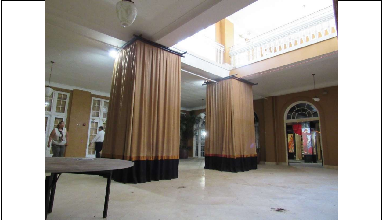
Photo #17 Gulfstream Hotel Building 1 Lake Ave, Lake Worth, FL 33460 Lobby area facing NE (11/7/2019)
