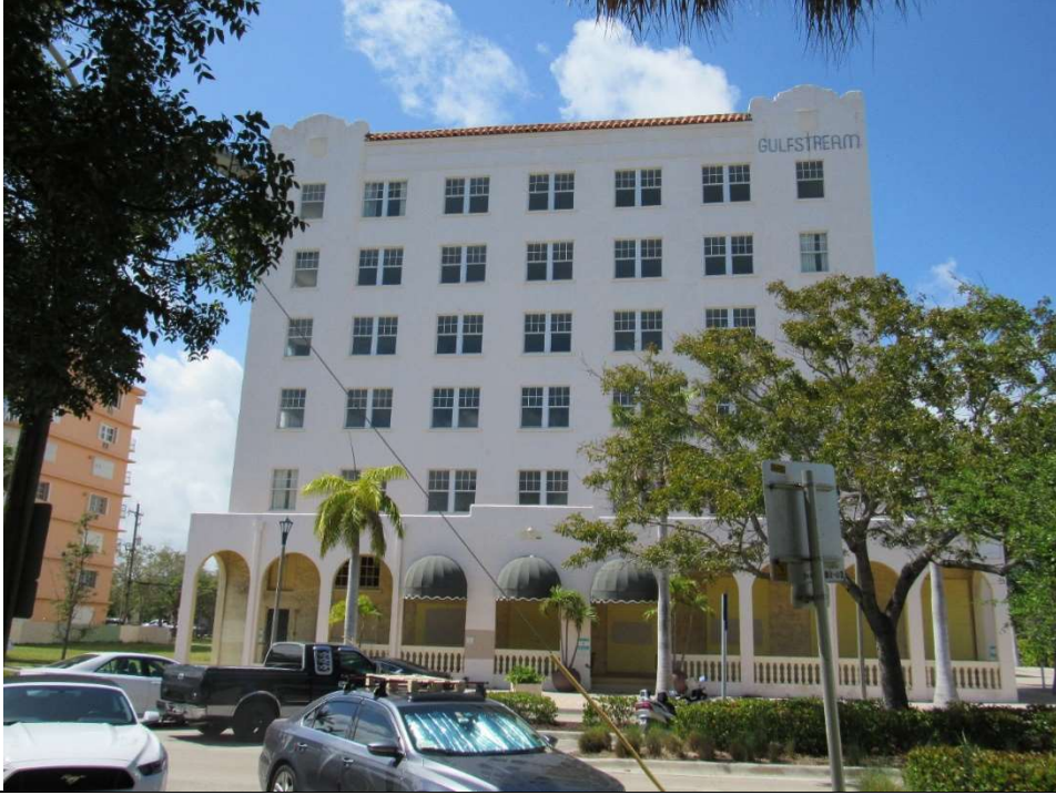
Photo #9 Gulfstream Hotel Building 1 Lake Ave, Lake Worth, FL 33460 View of entrance on E elevation (3/12/2020)
