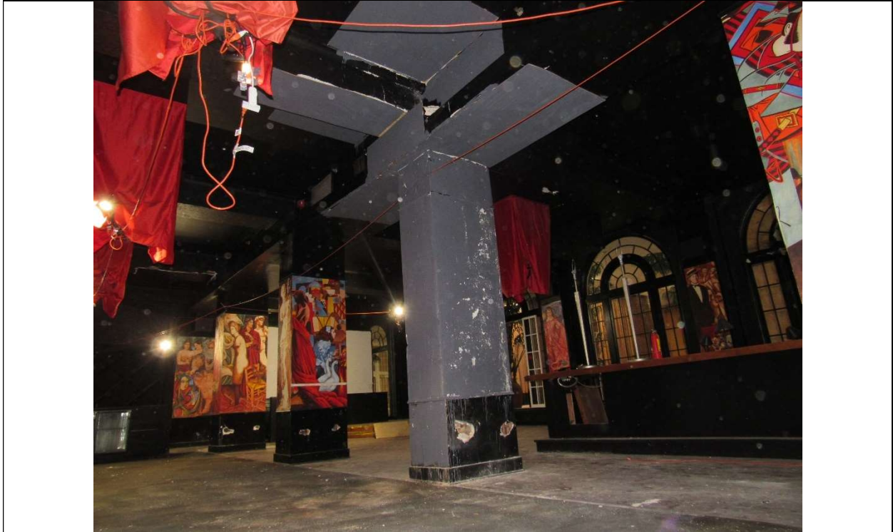
Photo #29 Gulfstream Hotel Building 1 Lake Ave, Lake Worth, FL 33460 E wing facing SW (11/7/2019)
