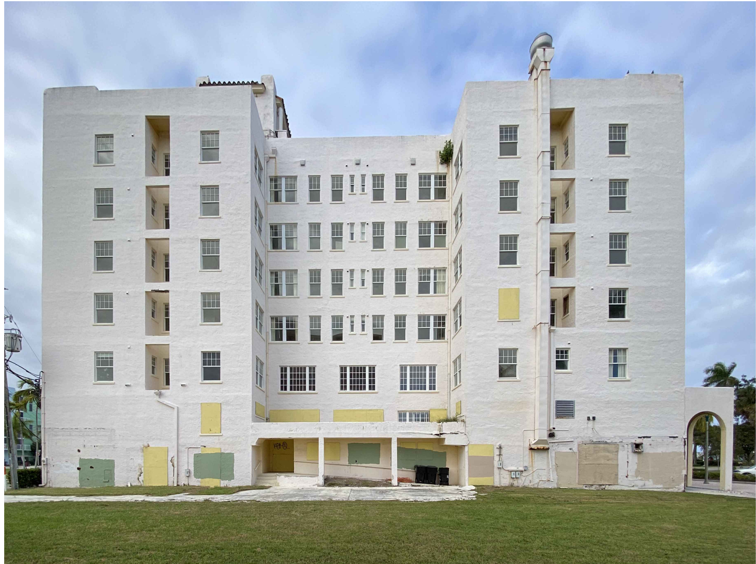
EXISTING BUILDING LOOKING NORTH
