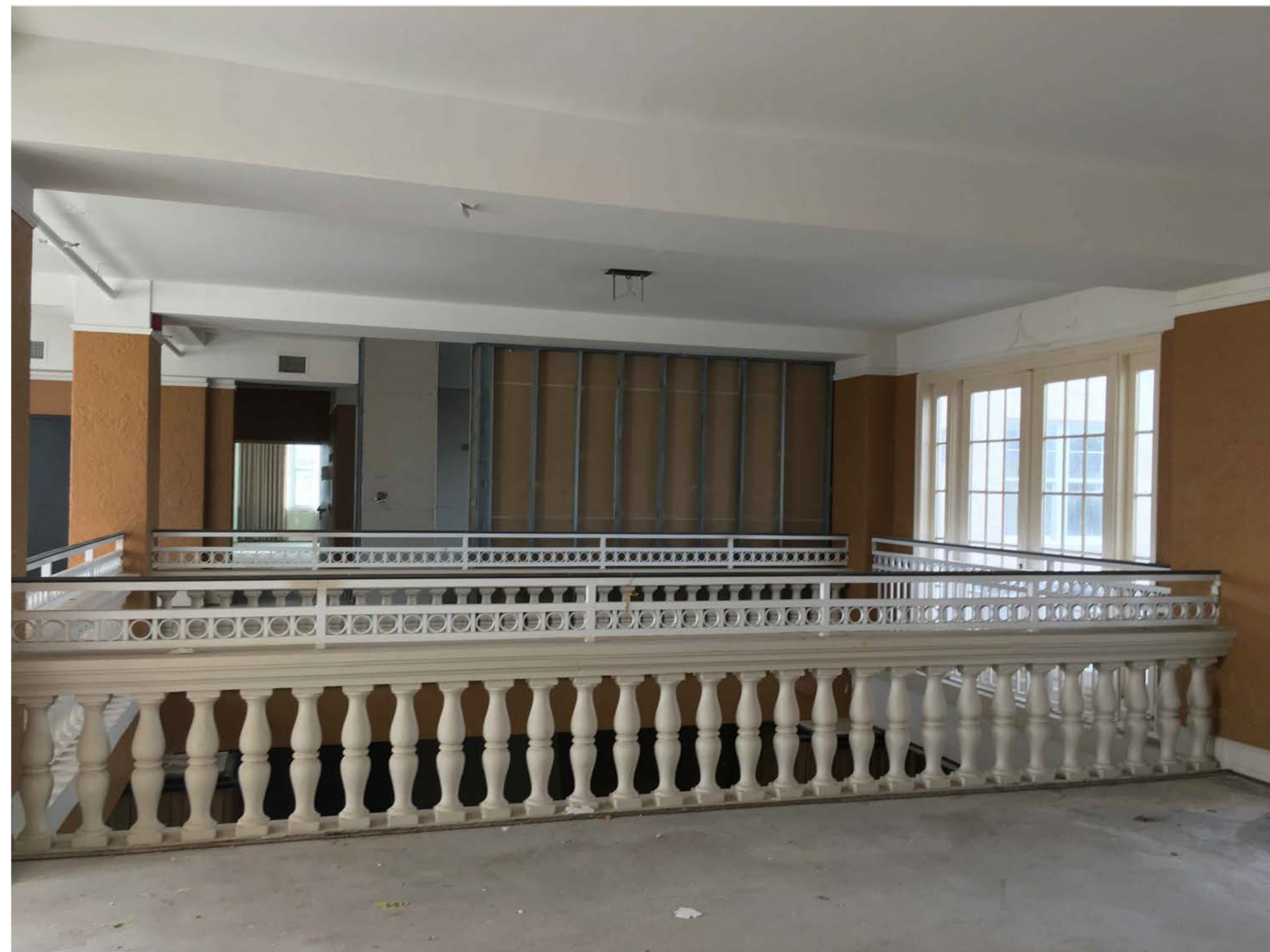
INTERIOR PRECAST CONCRETE RAILINGS
