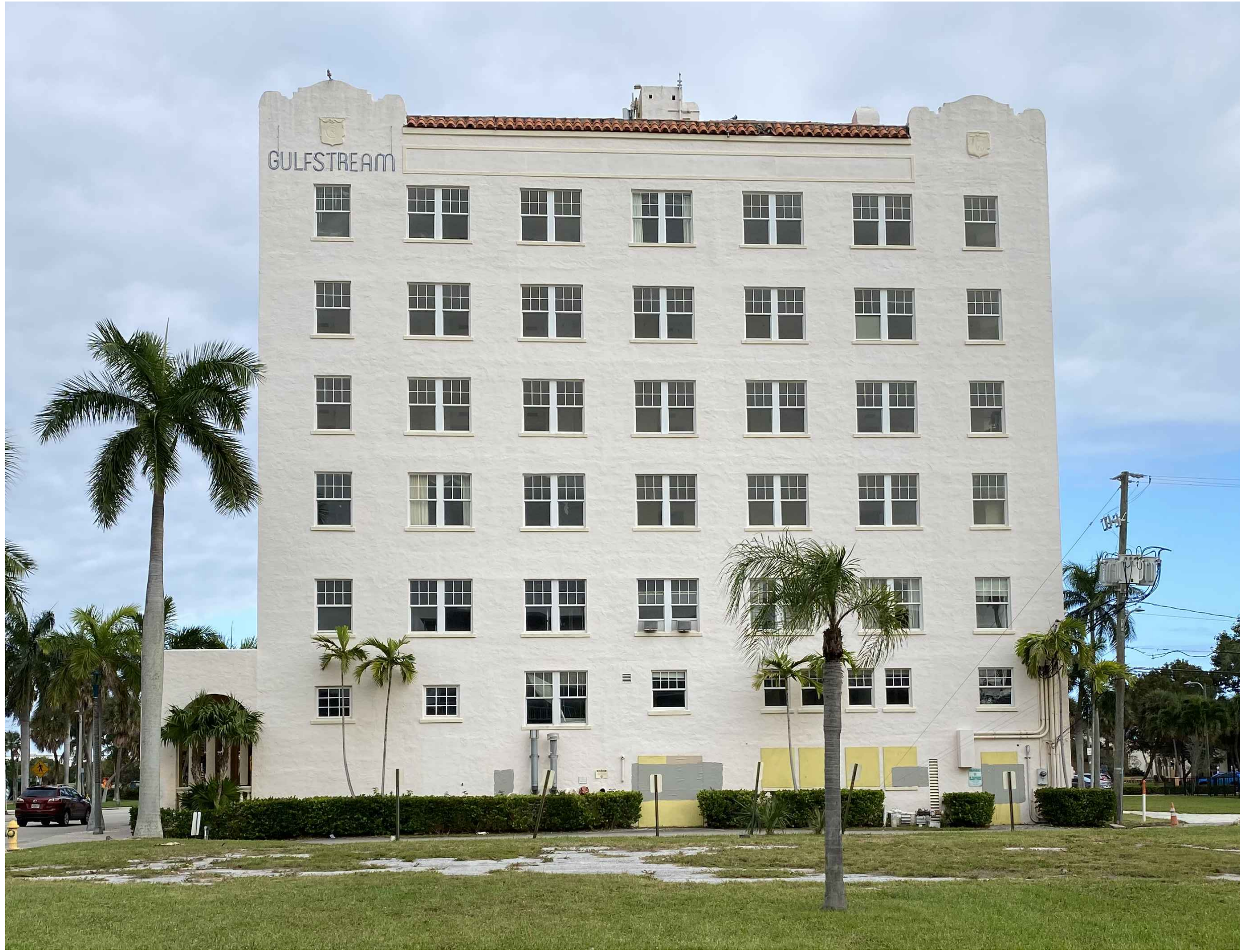
EXISTING BUILDING LOOKING EAST
