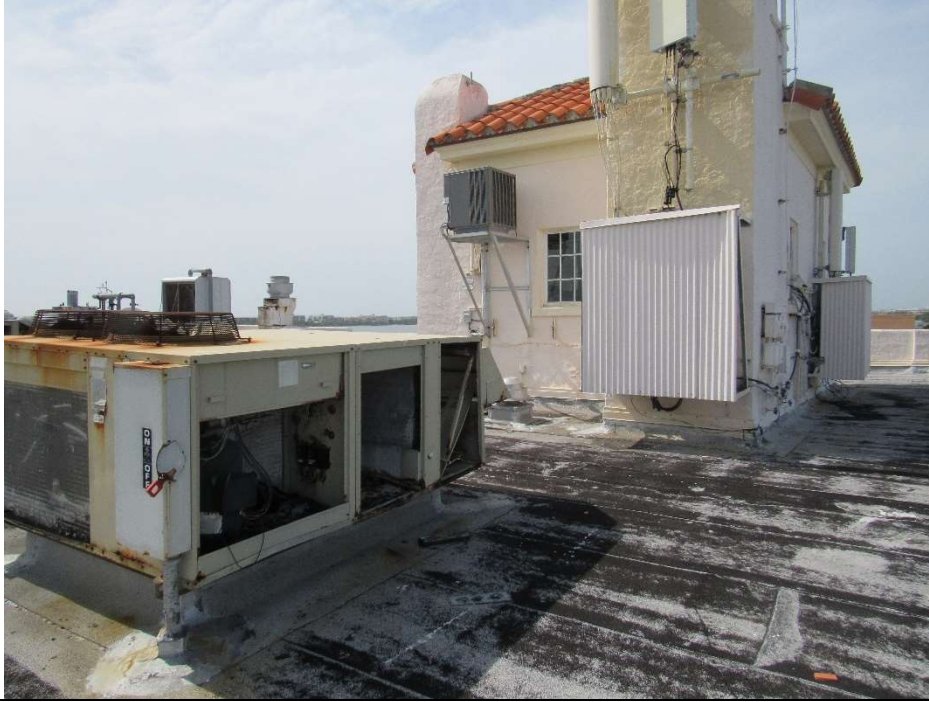
Photo #76 Gulfstream Hotel Building 1 Lake Ave, Lake Worth, FL 33460 Rooftop (7/10/2020)
