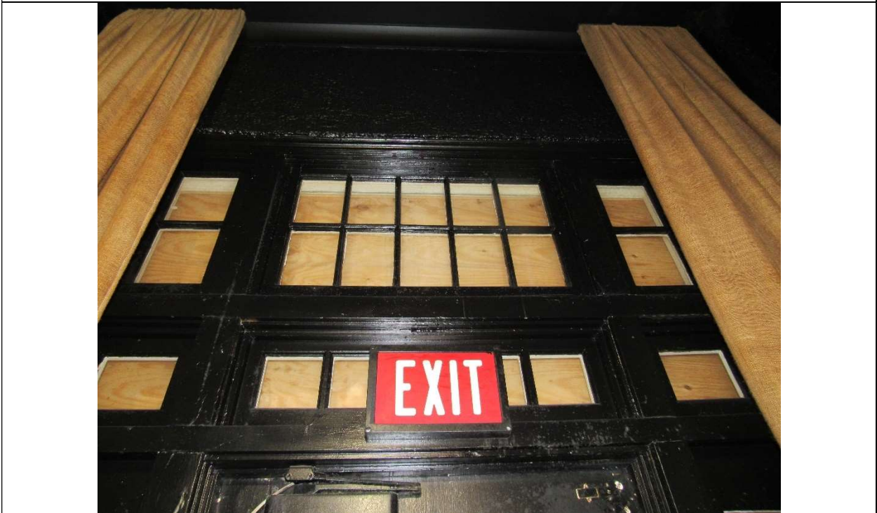
Photo #32 Gulfstream Hotel Building 1 Lake Ave, Lake Worth, FL 33460 Close-up of original exit doors in east wing (boarded from exterior) (11/7/2019)
