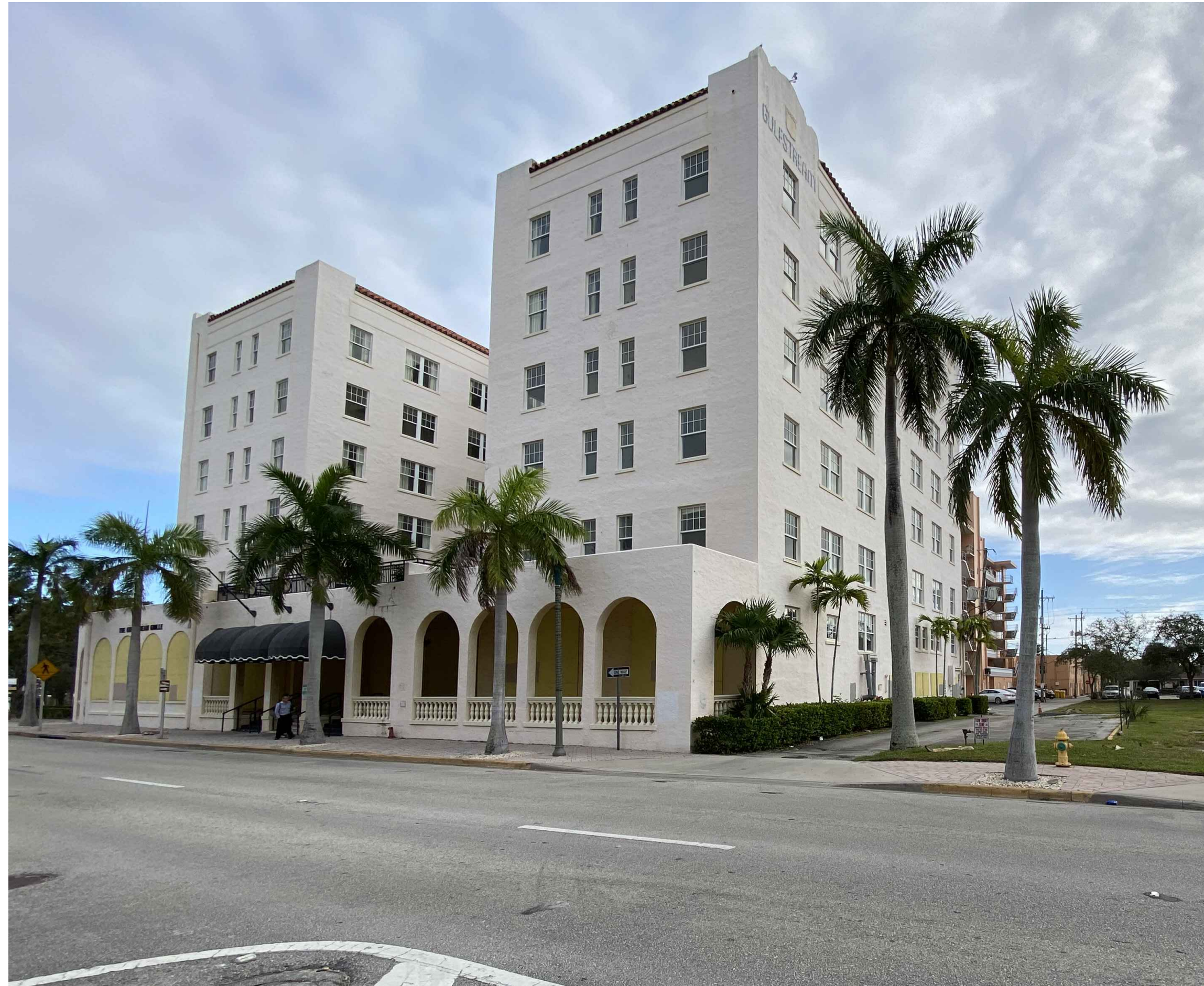
EXISTING BUILDING LOOKING SOUTHEAST
