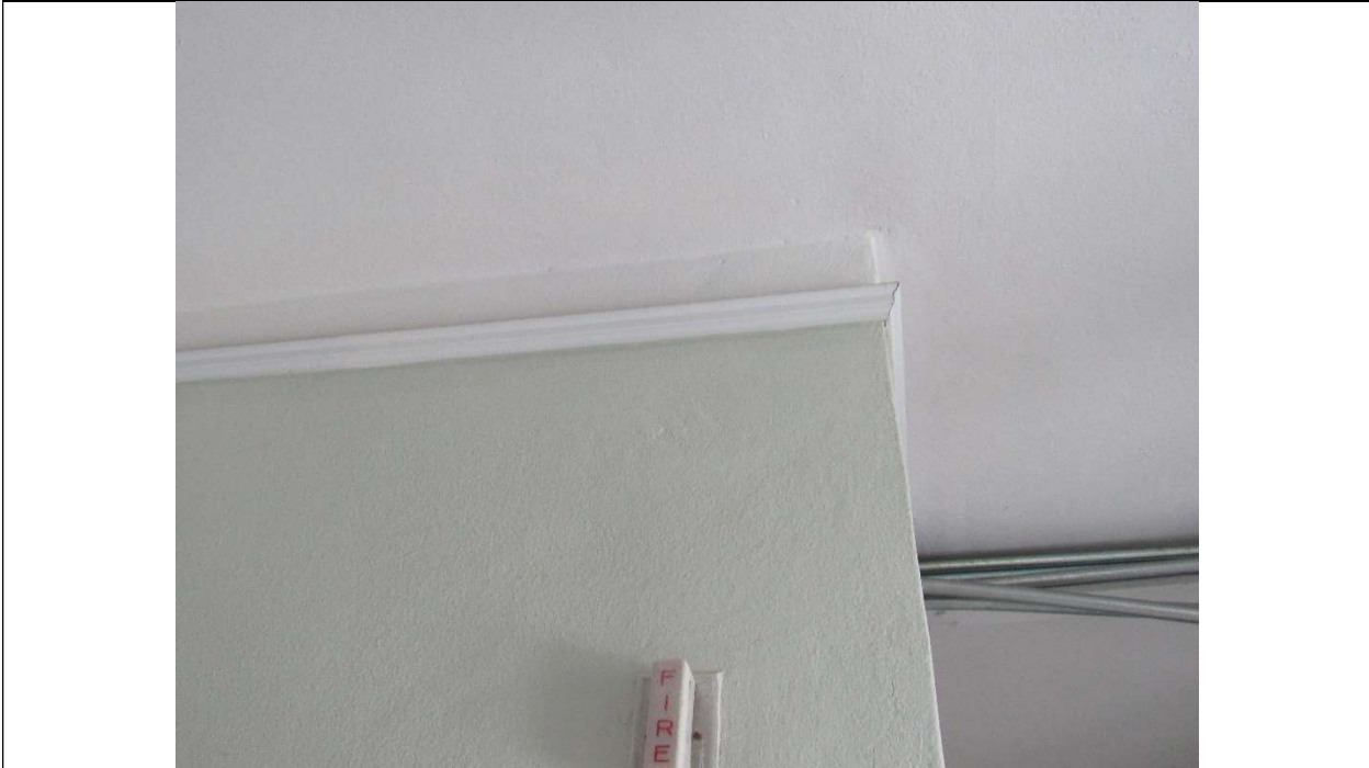
Photo #55 Gulfstream Hotel Building 1 Lake Ave, Lake Worth, FL 33460 Close-up of crown molding – third floor (7/10/2020)
