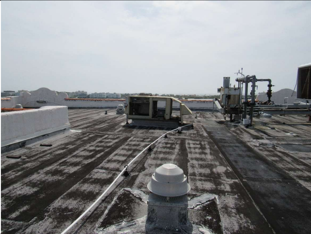
Photo #77 Gulfstream Hotel Building 1 Lake Ave, Lake Worth, FL 33460 Rooftop (7/10/2020)
