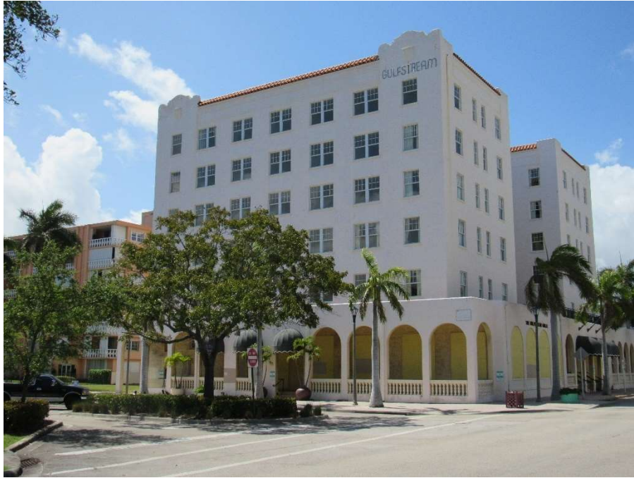
Photo #1 Gulfstream Hotel Building 1 Lake Ave, Lake Worth, FL 33460 View of NE Corner of Building (3/12/2020)
