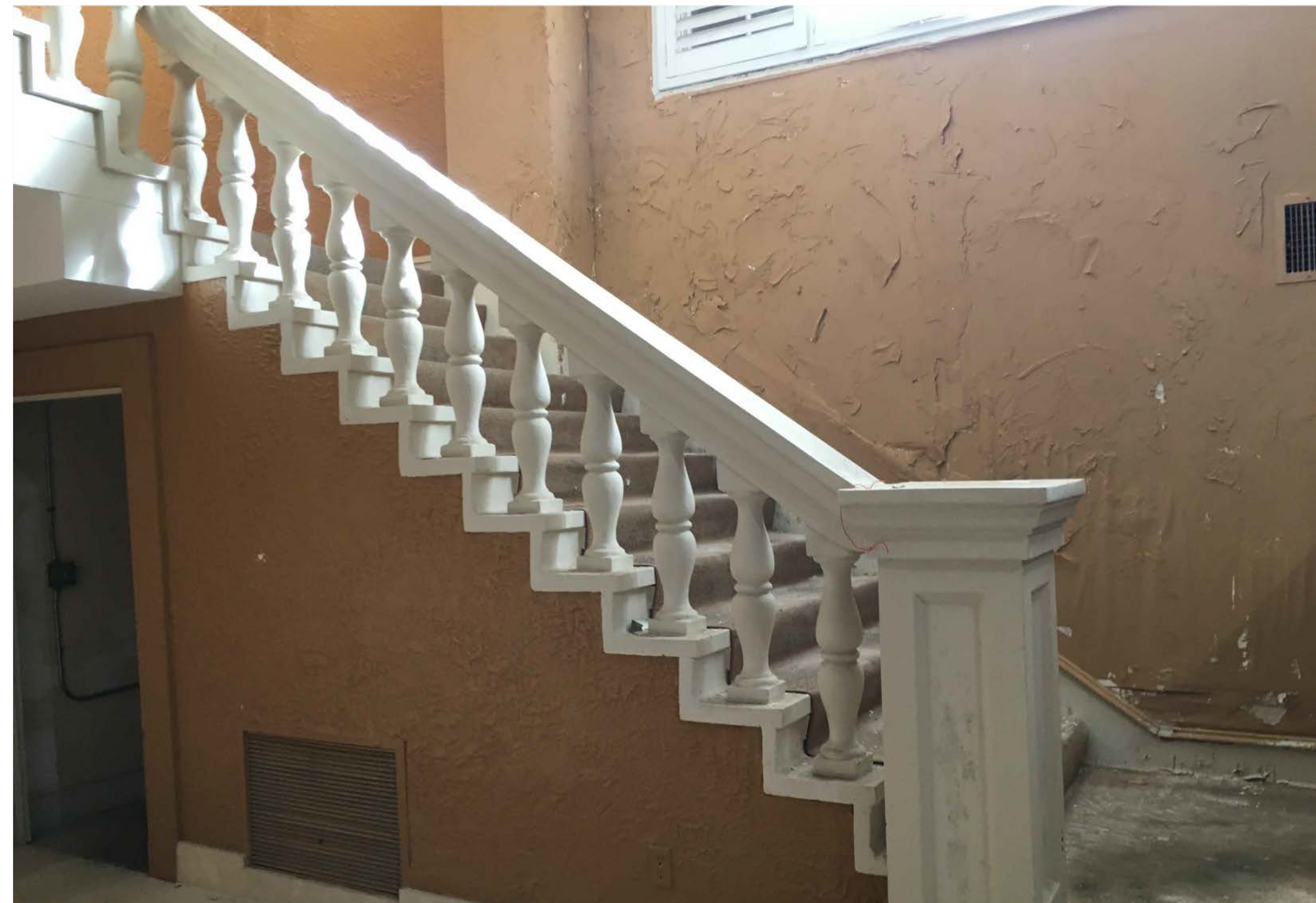
INTERIOR PRECAST CONCRETE RAILINGS
