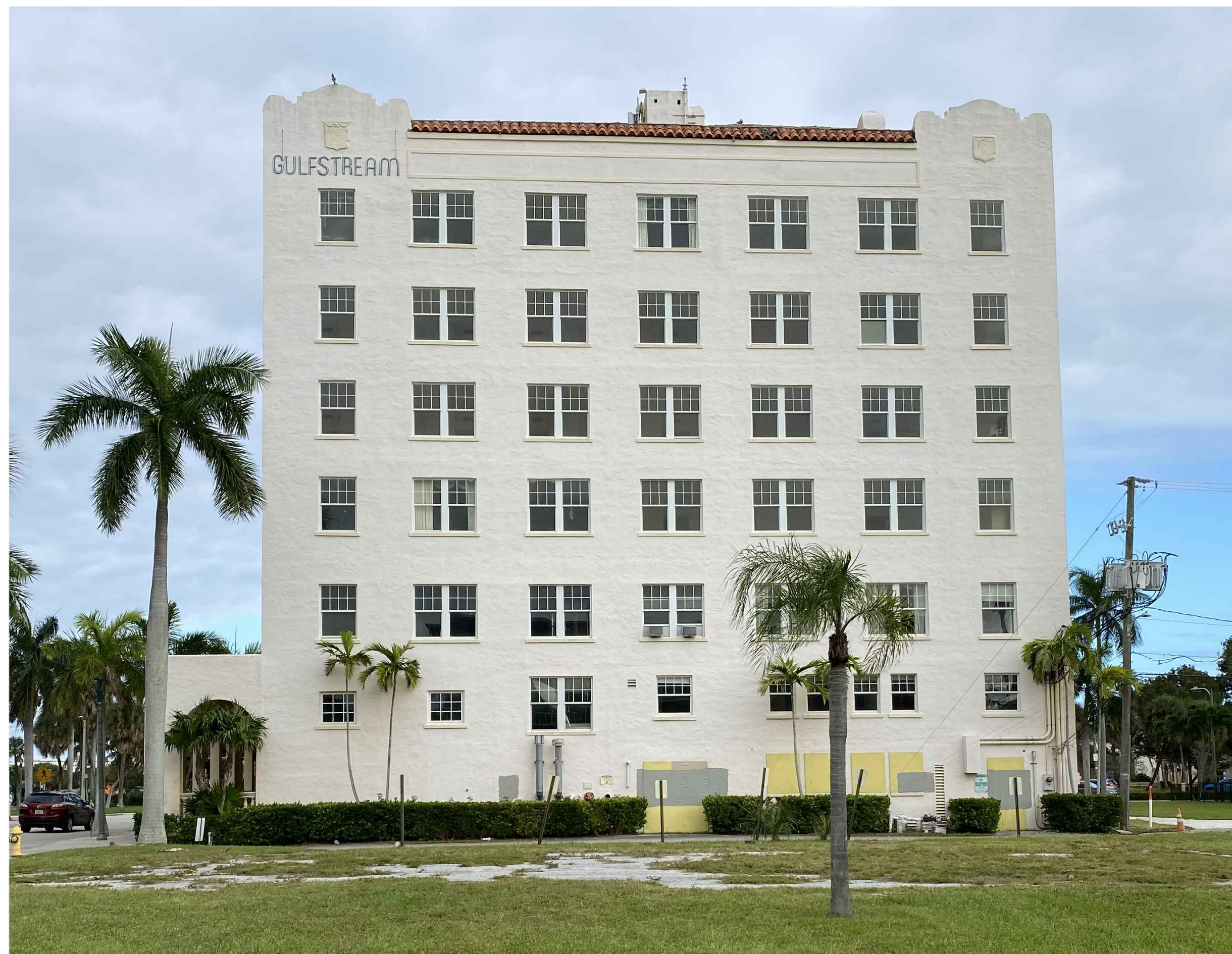
EXISTING BUILDING LOOKING EAST ARCADE, DECORATIVE PARAPET, TRIMS, RAILINGS, TILE ROOF, SHIELDS AND SIGNAGE TO REMAIN. EXISTING WINDOWS AND DOORS TO BE REPLACED WITH NEW WINDOWS AND DOORS (MULLION CONFIGURATION TO MATCH EXISTING)
