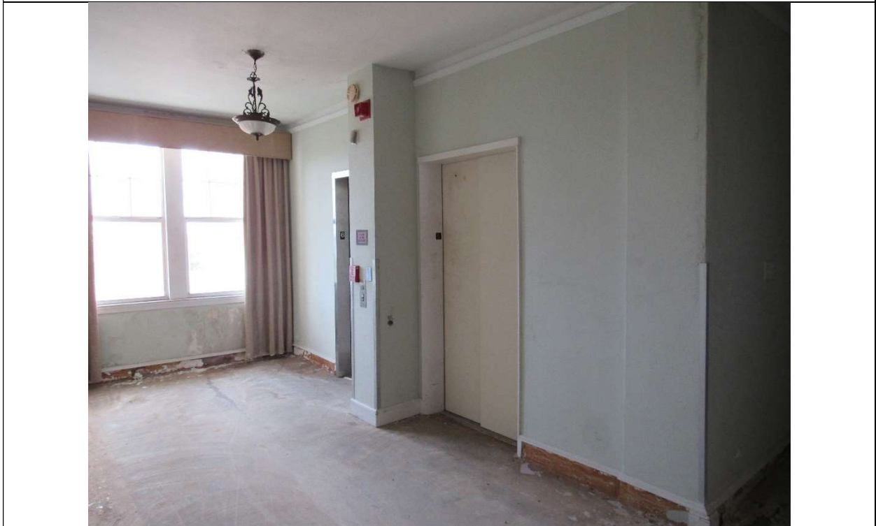
Photo #69 Gulfstream Hotel Building 1 Lake Ave, Lake Worth, FL 33460 Sixth floor elevator lobby (7/10/2020)
